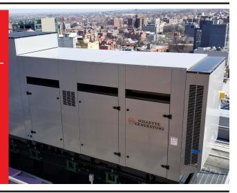
This project involves a 250KW Standby diesel generator, the SPVD-2500 Volvo powered standby diesel generator fit the need. The project was for a high-rise hotel installation in Flushing, NY. There are many layers of codes, restrictions and requirements in the power generation industry, primarily the NYC Rooftop code.
