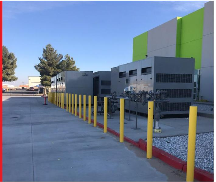
In 2019 Gillette Generators provided 10ea. PR-5400, 540KW prime rated natural gas generators utilizing PSI's proven heavy duty 32 liter engine, Stamford Generator end, Basler HD 2020 Synchronizing controllers, and ABB motorized circuit breakers for a large cannabis customer in Southern California.
