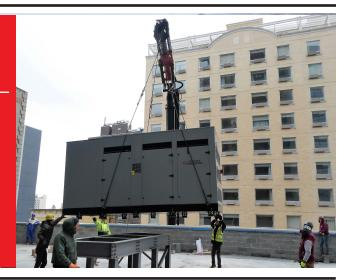
This was a urgent need for a quick turn-around on a 500kw Standby diesel generator, Our SPVD-5000 Volvo powered standby diesel generator fit the need. The project was for a high- rise hotel installation in Long Island City, Queens, NY.
